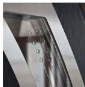
Triple-glass packets with Super Spacer bar
